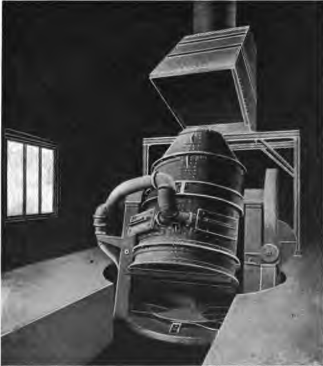
FIG. 234.—Stock Converter. Blowing Position.
